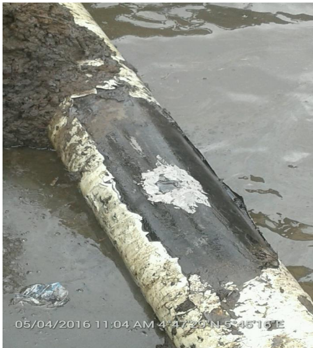
10" pipe still intact
